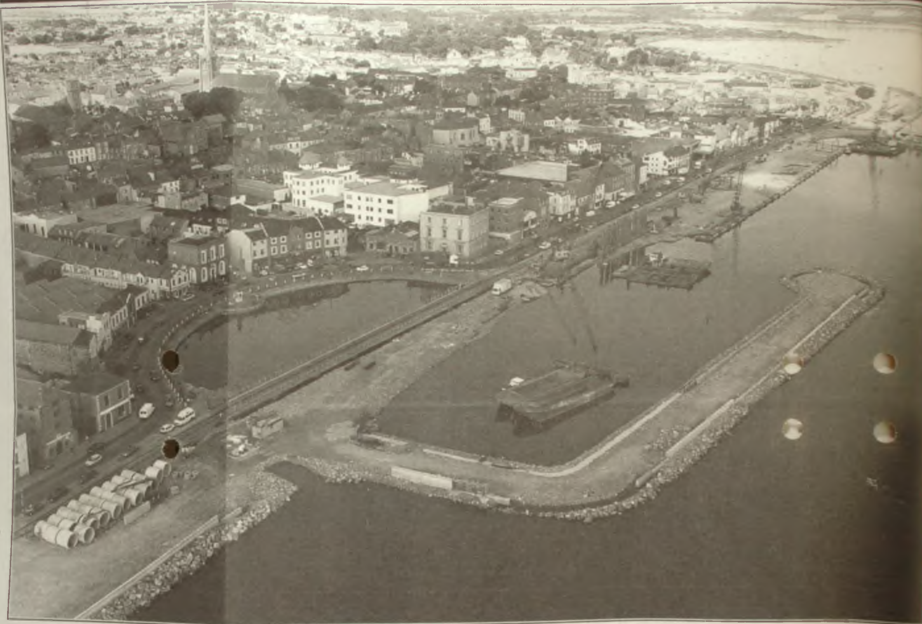
■ An aerial view of Wexford Harbour with work on the marina in progress.
